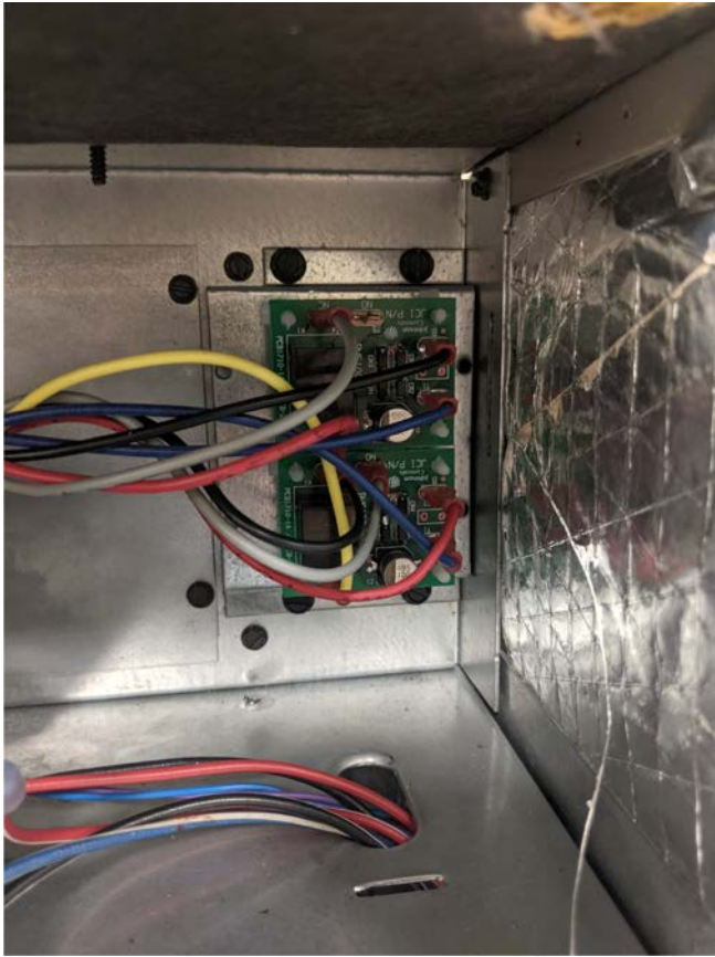
Figure 1: Air handler relay plate installation
